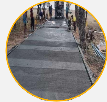
RCC Flooring Road
