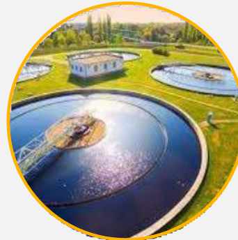
West Water Treatment Plant
